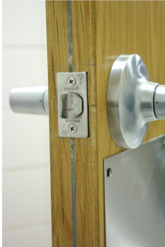
*Figure 2.7.2.1: Example of lead-shielded door with lead layer visible in the center of the door slab. (Image used with permission from RAD-Planning)*
